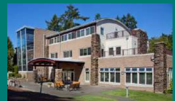
ARCHBISHOP BRUNETT RETREAT CENTER AT THE PALISADES Federal Way, WA
